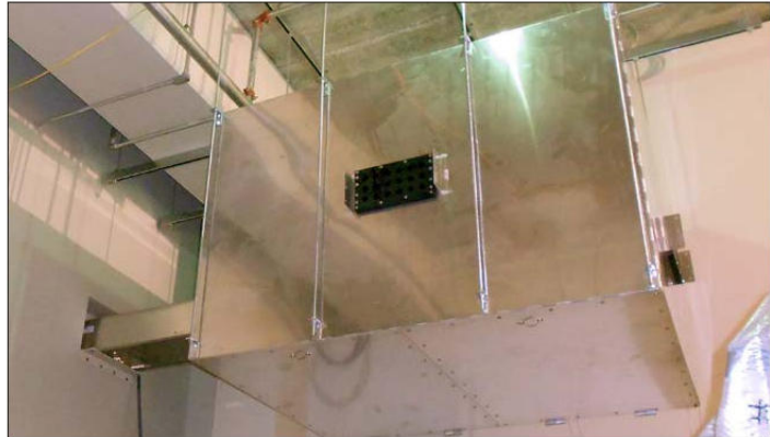
RIGHT—Installed Cable Bus system featuring a custom tap box .
